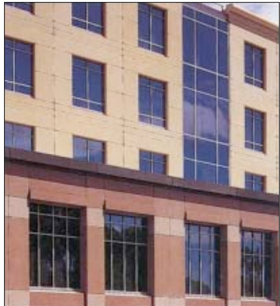
Panel-to-panel joints and false joints articulate the cream GRC cladding and the reconstituted granite podium cladding at St George Private Medical Complex Kogarah NSW
